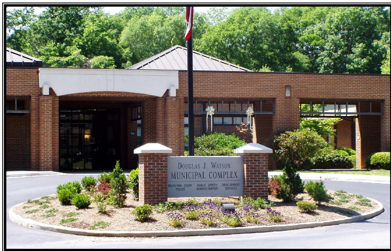
Pictured: The municipal buildings on North Ross Street were rededicated in honor of Dr. Douglas J. Watson, a respected community leader who retired in 2003 after serving as Auburn's City Manager for over 20 years.
