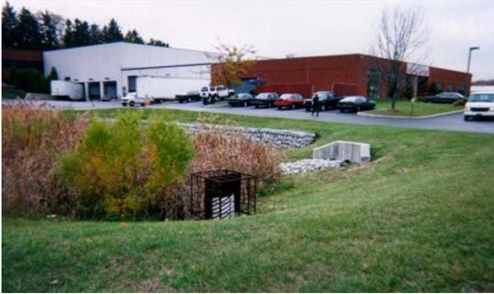
FIGURE 4-29 Dry Extended Detention Basin with Shallow Marsh
