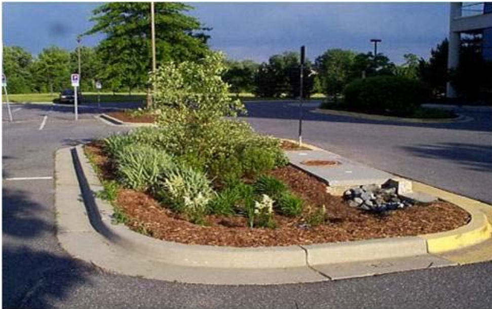
FIGURE 4-3 Bioretention in Parking Lot Island
