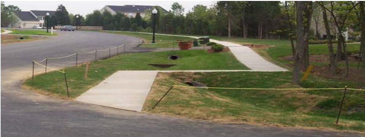
FIGURE 4-9 Recently Constructed Grassed Swale in Residential Area, Pembroke Woods Subdivision in Emmitsburg, MD (Courtesy of Mike Clar, Ecosite, Inc., Columbia, MD)
