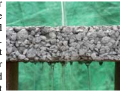
Permeable Pavement Cutout
